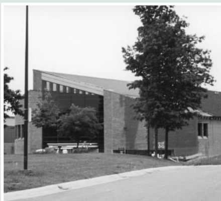
A new entrance to Building A at Orchard Ridge helped visitors and students identify this key building.
