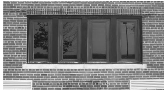
Lintel tuckpointing, High Oaks Hall
