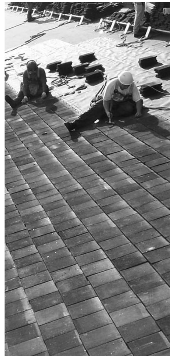
Clay tile roof replacement
