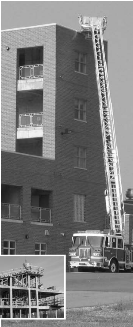
CREST fire training structure from construction to completion
