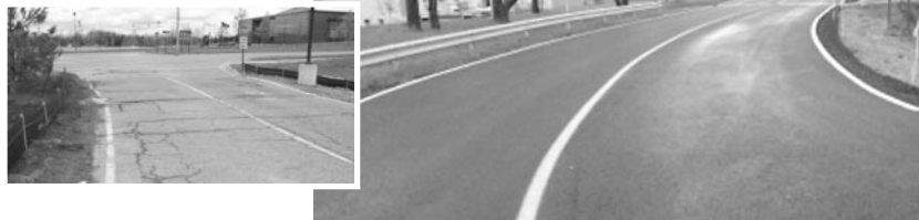
College-wide road and sidewalk repair and replacement programs
