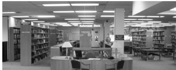
Building D second-floor renovations
