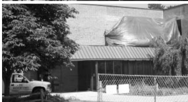
Masonry flashing and roof panel repairs
