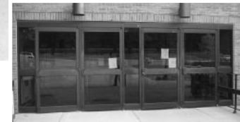
Exterior door replacements
