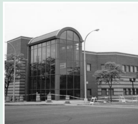
The new wing at the Royal Oak Campus was designed to house computer labs and computer-assisted classes, as well as a child-care facility.
