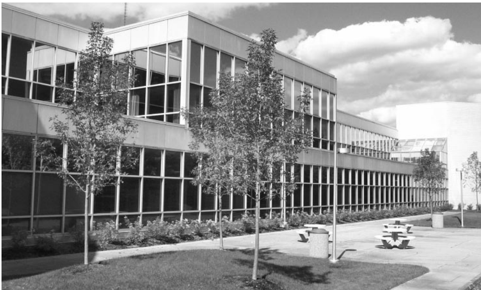
Exterior aluminum curtainwall replacement
