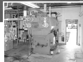
Boiler, electrical replacements at District Office
