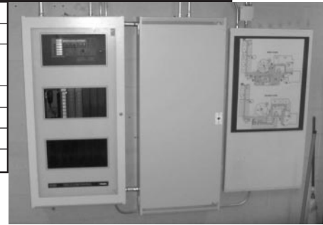
Fire alarm upgrades
