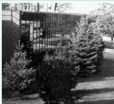
The new power plant at the Highland Lakes Campus has provided the campus with energy efficiently.
