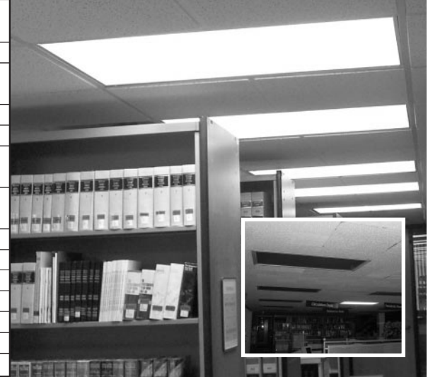
Ceiling and lighting replacements, Building K
