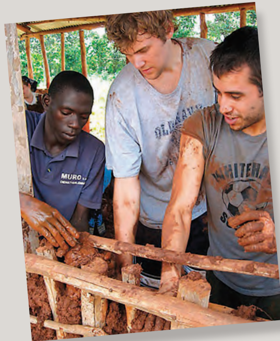
▲ Uganda interns Mike Upshur and Patrick Nulty assisted with the creation of mud walls for a new church building during their 2006 visit to Africa.
