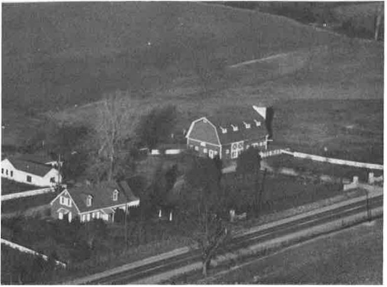
Aerial view of recently acquired 54 acre campus addition
