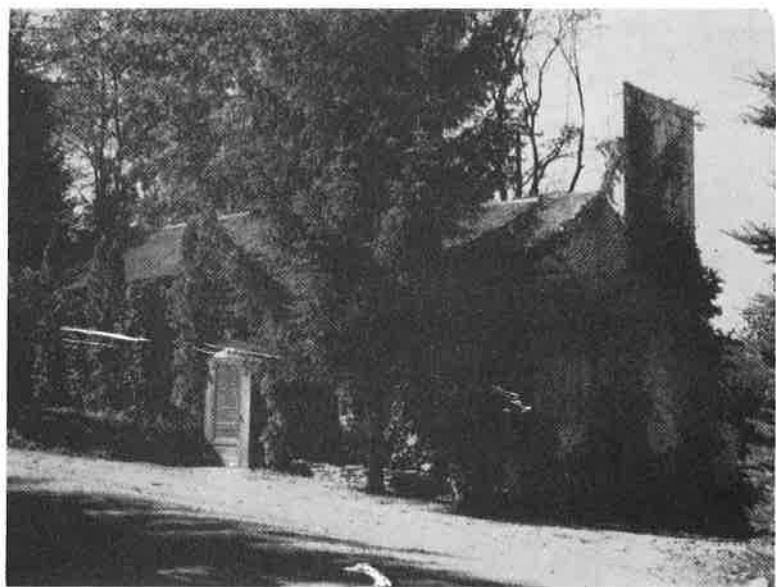
Maintenance Supervisor's House
