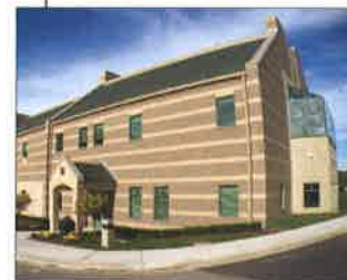
Richardson Center completed
