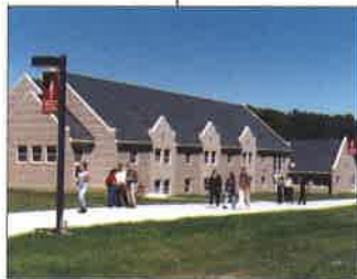
Ferndale-Hoggatt Hall completed
